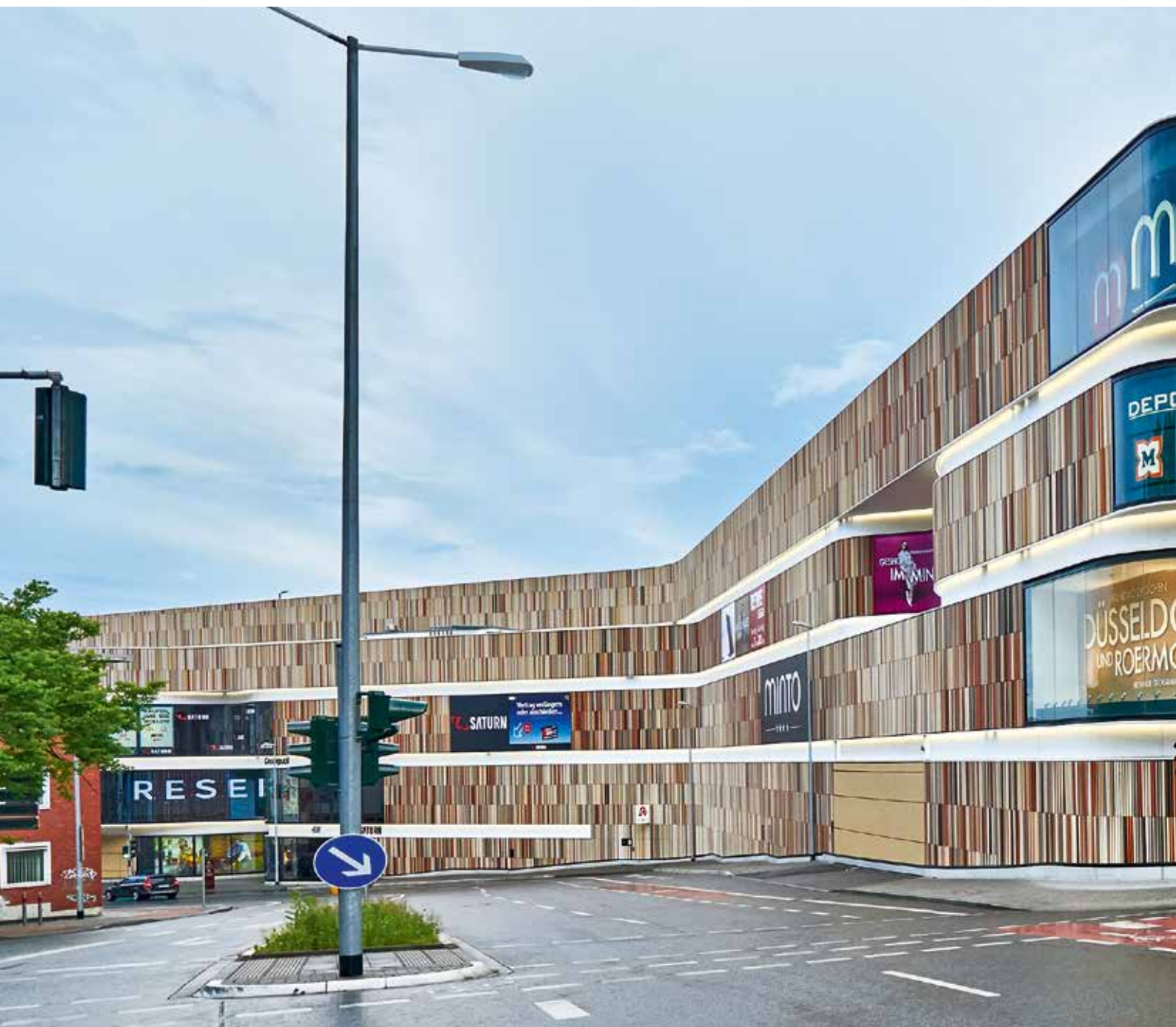
The powerful facade creates a new centre for Mönchengladbach. The advertising spaces are integrated and not only placed on top.
