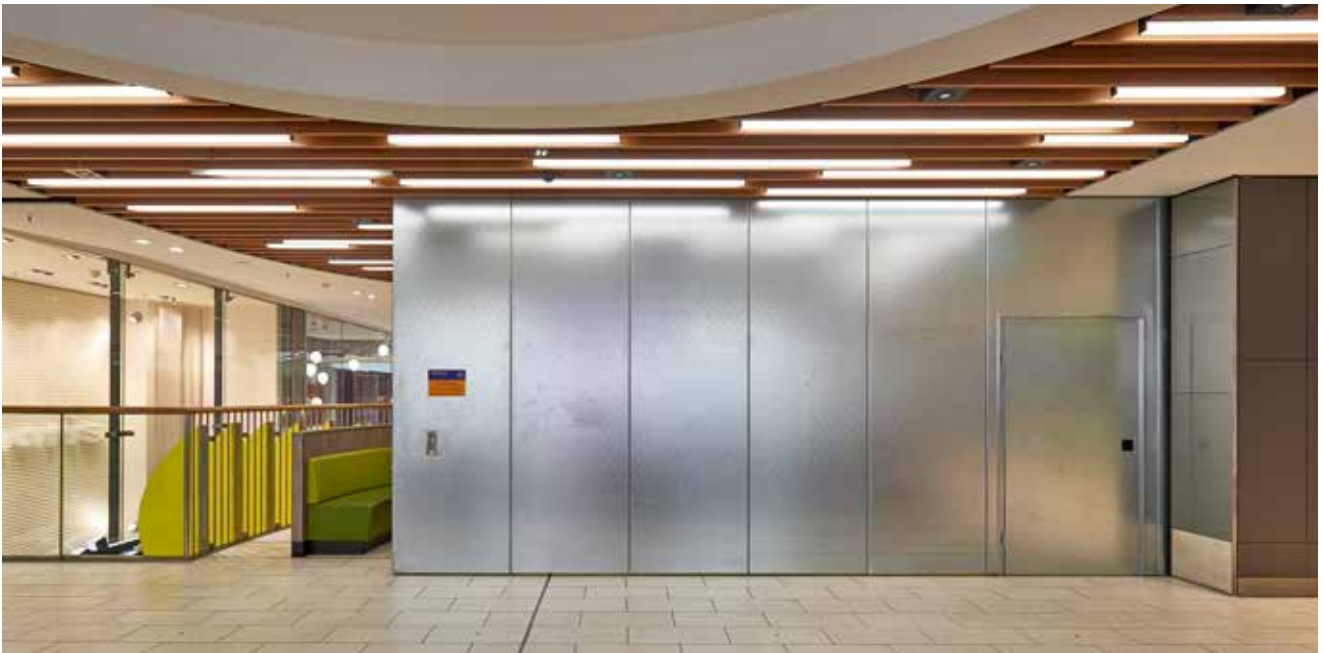
In case of fire, fire sliding doors extend from the wall to separate the individual fire protection zones from each other.
