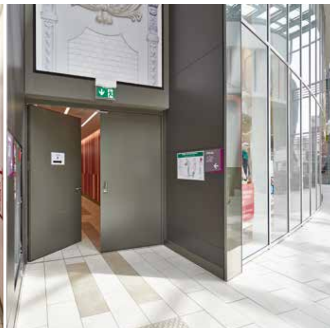
External door with ventilation slats. Double-leaf fire-rated and smoke-tight doors protect the escape routes to the outside.
