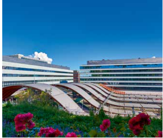
The sweeping roofs of the platforms are still under construction.
